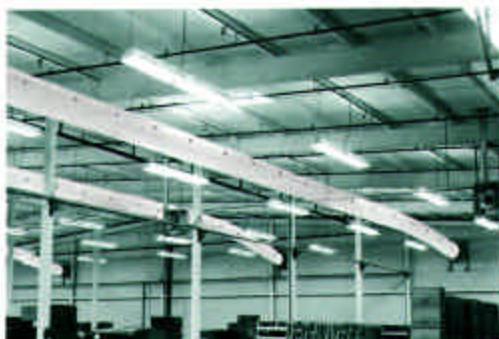
FAN-JET® does its job near the roof, mixing cold make-up air with heated ceiling air.
